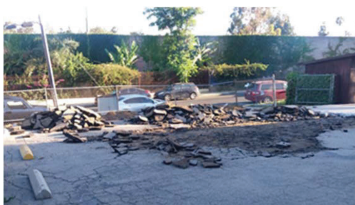
Repaving parking lot Summer/2017
